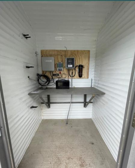
For measuring water level, the most common method is with a bubbler and pressure sensor. The recorded values are logged every 15 minutes on an on-site data logger and transmitted out via satellite once an hour. Currently we use the FTS bubbler, though there was a manufacturing defect that caused a great deal of lost data and consternation, and is still slowly being addressed.
