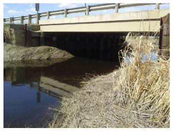
Photo No.: Photos-20180507-202135.jpg Description: Sediment Erosion
