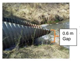
Photo 1: Culvert outlet gap at WC\_0772 located on Highway 16 over Atim Creek.
