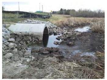
Photo No.: Photos-20180509-213309.jpg Description: Inlet / Erosion
