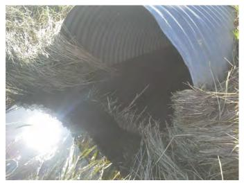
Photo No.: Photos-20180507-162947.jpg Description: Culvert 1 - Blockage In
