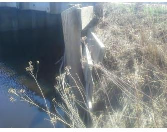
Photo No.: Photos-20180508-190608.jpg Description: Wing Wall Damage
