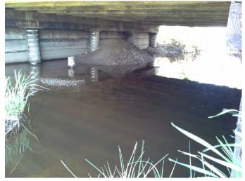
Photo No.: Photos-20180518-151547.jpg Description: Sediment buildup
