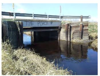
Photo No.: Photos-20180507-191928.jpg Description: Outlet & Wingwall condition-materials falling
