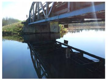
Photo No.: Photos-20180511-171930.jpg Description: Erosion under abutment
