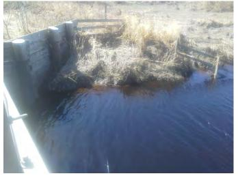
Photo No.: Photos-20180508-184851.jpg Description: Erosion Ditch Slumping
