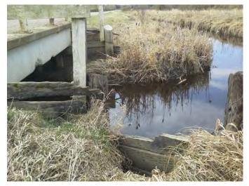
Photo No.: Photos-20180509-173431.jpg Description: Wing wall damage and lack there of wingwall as well rotting on east side top
