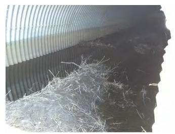
Photo No.: Photos-20180507-194508.jpg Description: Bank slump in culvert
