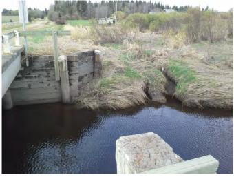
Photo No.: Photos-20180509-182050.jpg Description: Increasing sedimentation around wing walls
